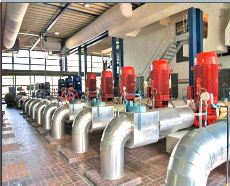
PUMPS INSTALLED IN STEEL PLANT
